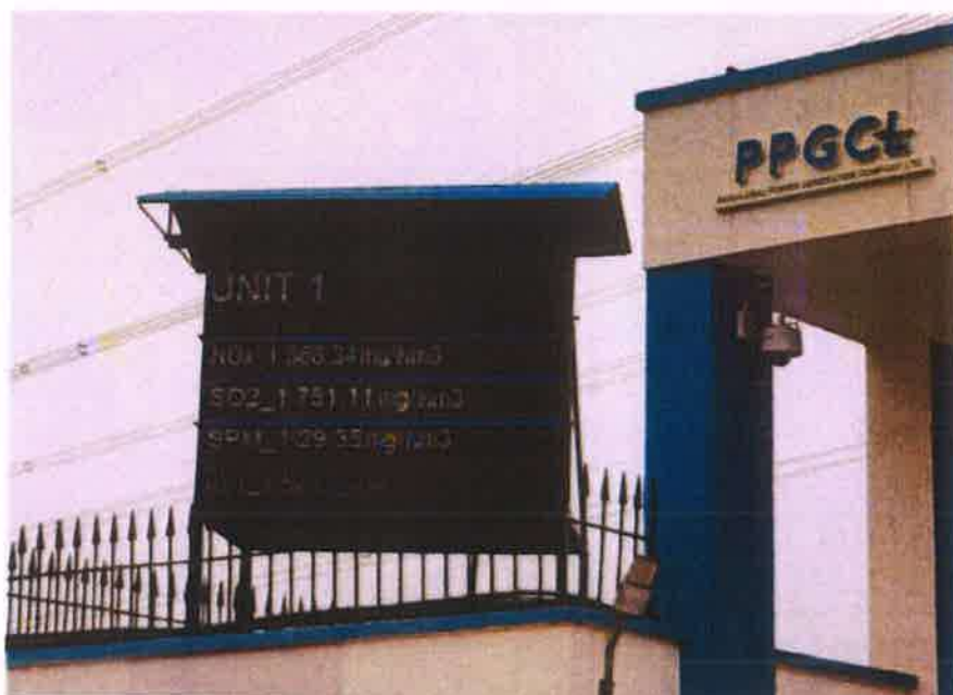
Data of Stack and ambient air display at main gate of the Plant
