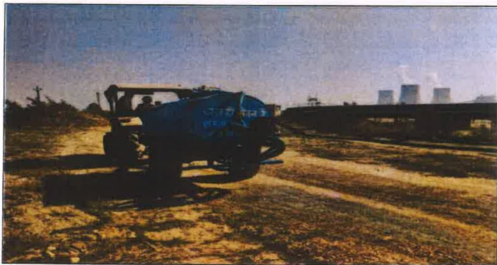
Water sprinkling through tankers in ash pond bund
